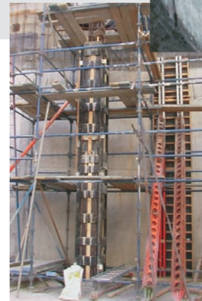
500mm x 500mm x 9 metres tall IN-SITU COLUMNS
